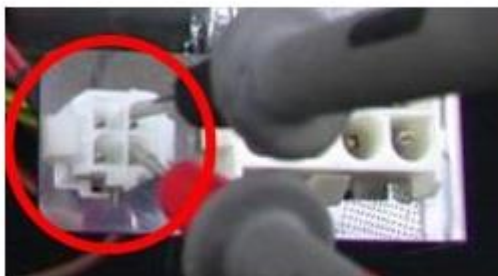
NTC sensor Boiler 1
